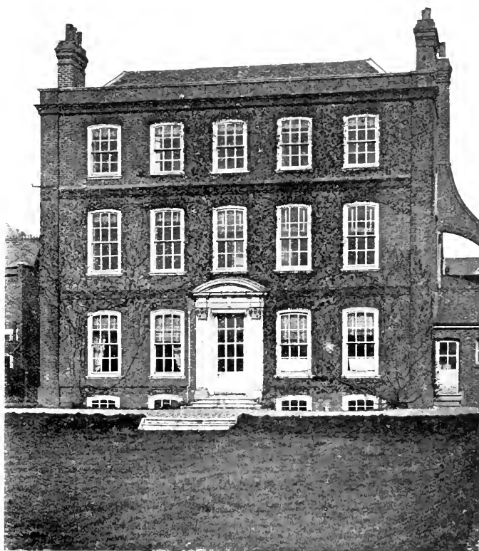
226. Friends' House, Croydon. Garden Front.
